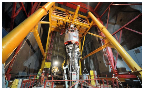
Shaft sinking operations
